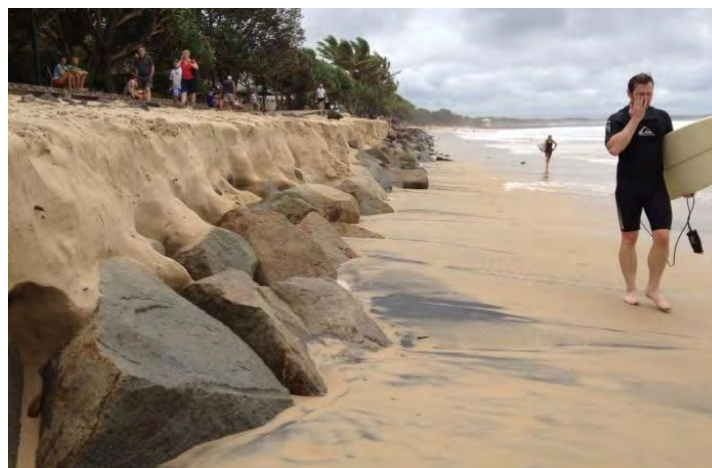
Steep Erosion Cliffs
